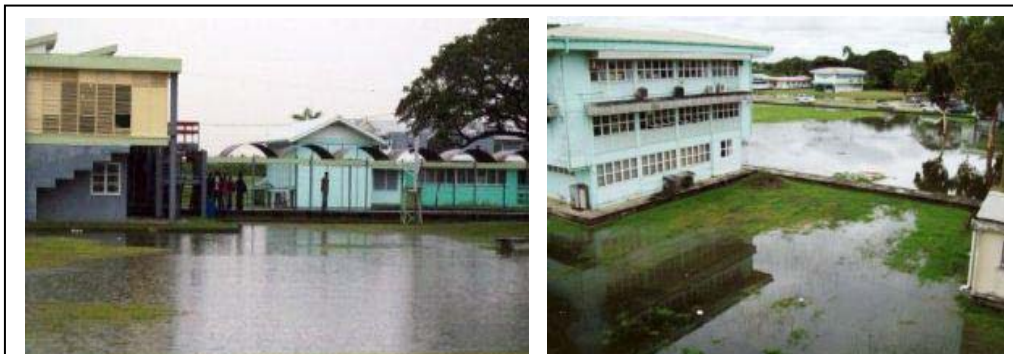
Figure 9 Flooding of the University of Guyana Turkeyen Campus, after a heavy rainfall
