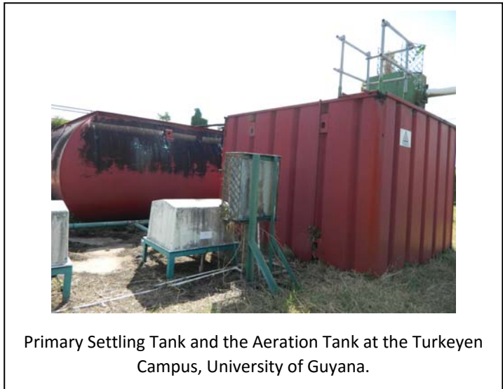
Figure 17 Settling and Aeration Tanks
