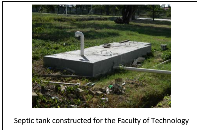
Figure 18 Septic Tank at the Faculty of Technology
